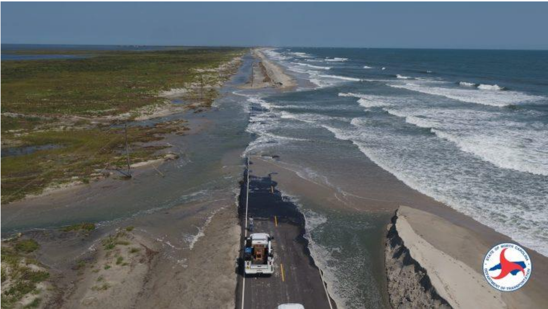
N.C. 12 on Ocracoke Island after September 2019's Hurricane Dorian: Photo: NCDOT
